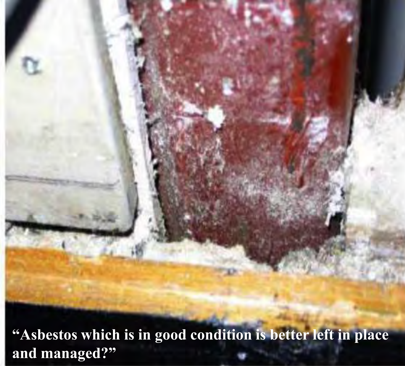
Figure 11: View of base of column from which the casing in figure 10 was removed. A large amount of friable AIB debris can be seen.
